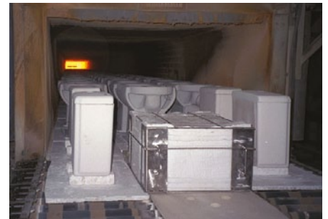
Kiln Tracker system in roller hearth sanitaryware kiln
